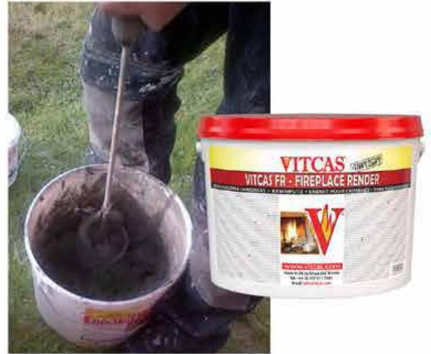
**1.** Coat the masonry with neat (undiluted) Vitcas PVA.
