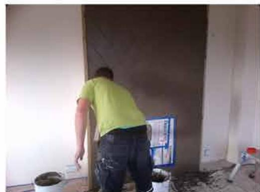
**5.** Use a straight edge between the two side guides to strike off the material.
